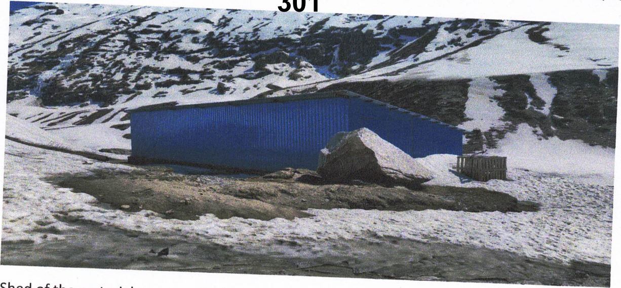
Shed of the material recovery facility.
