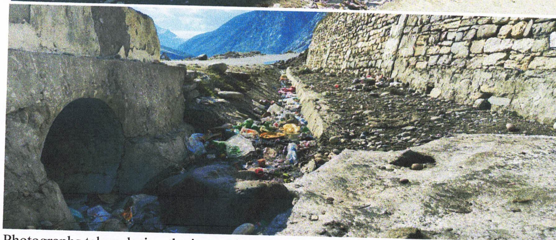
Photographs taken during the inspection on 21.05.2024.
