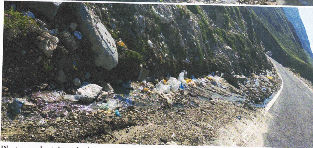
Photographs taken during the inspection on 20.07.2024.
